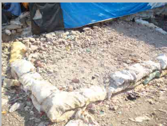
Figure 4.3. Land portion prepared for construction.
