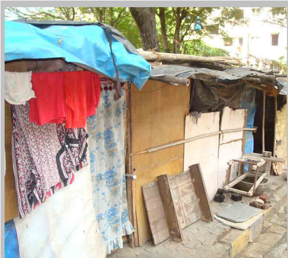
Figure 4.8. Housing condition in Sai Leela Pavement Dweller Community.
