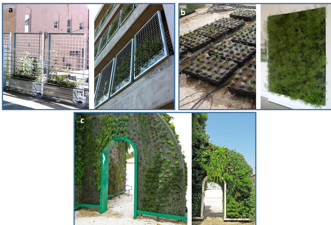
Figure 2.5.- Examples of green walls systems not rooted into the ground: a) Climbers rooted into containers; b) modular system and c) hydroponic system.
