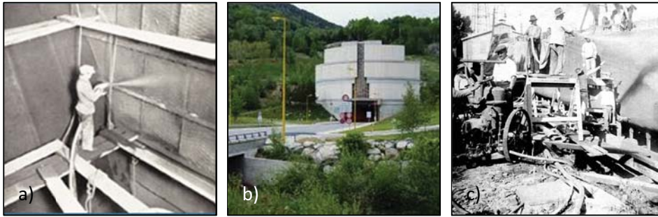
Figure 2.2- Protection of structures a) tunnel in Puymorens b) and construction of barges c)
