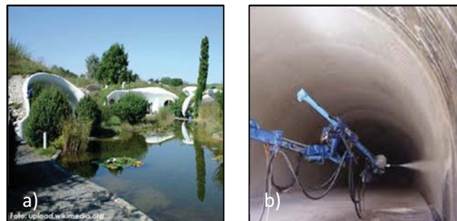
Figure 2.3- Sprayed concrete houses by Vetsch a) and spraying robots b)
