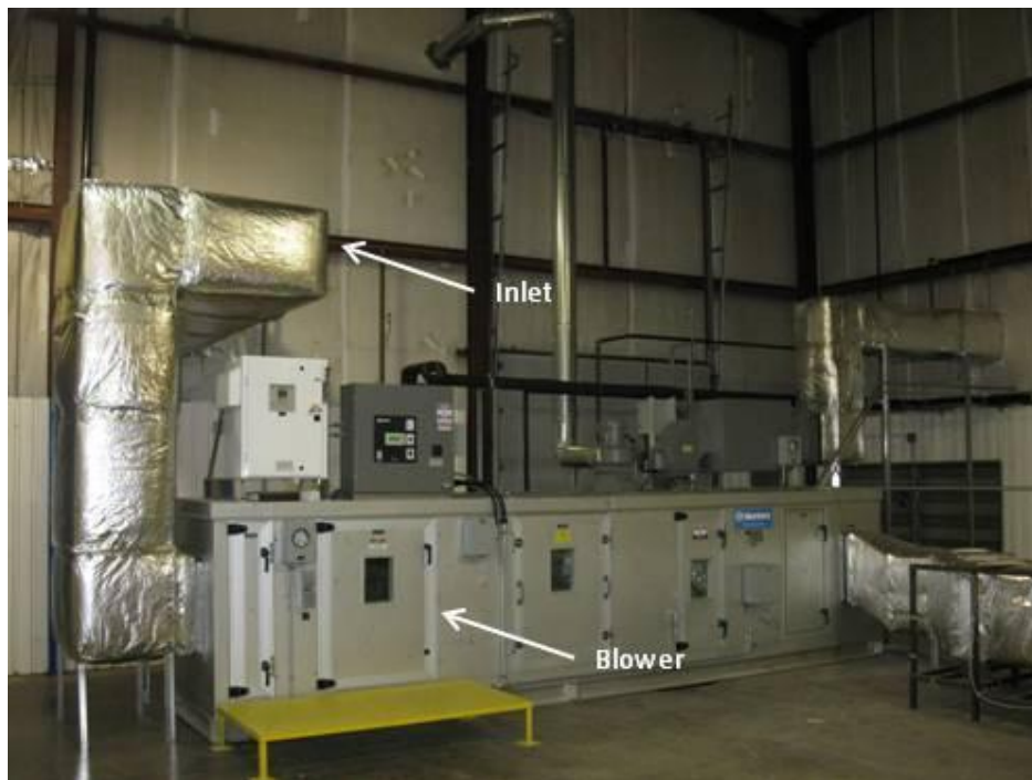
Figure 3.5 - Dehumidification system
