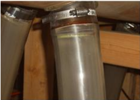
E) Hose Connection to Supply Duct
