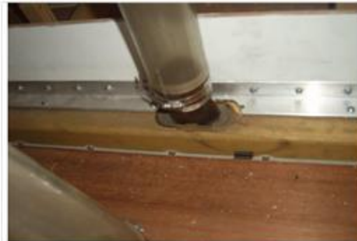
F) Hose Connection to Diffuser
