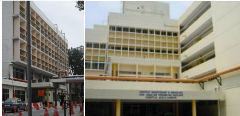
Figure 3: Shown the exterior of facade design at the RT building using concrete frame sun-shading overhang at the ward area
