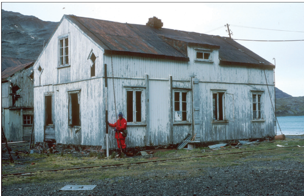
PLATE 4 The former Manager's Villa in Stromness where Ernest Shackleton and companions arrived in May 1916. Photo: D. Nevestad, NARE 89/90.
