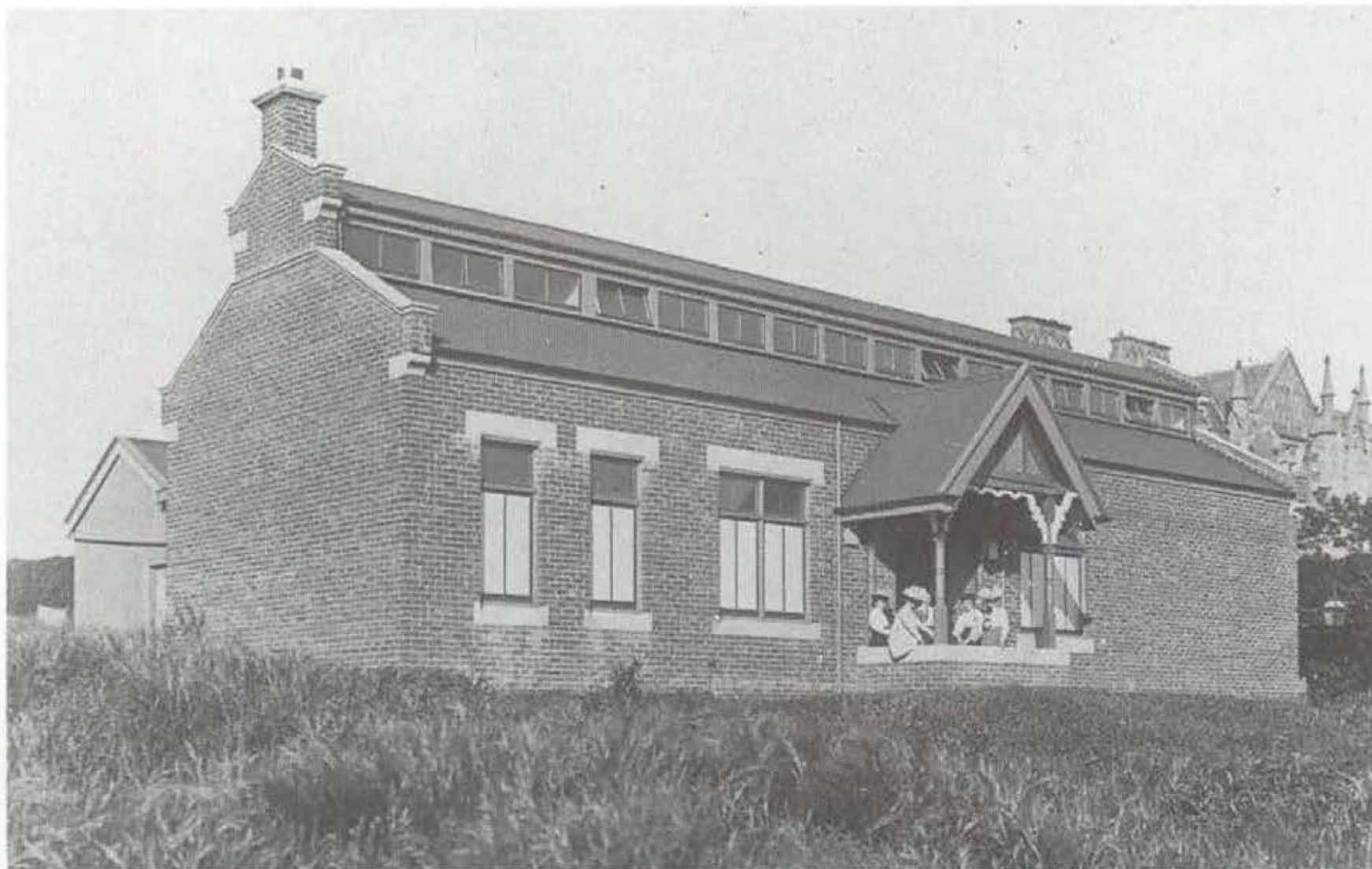
8. The Chemistry laboratory, in use from 1905. When Chemistry was moved to the Technical School in 1913, the laboratory was taken over by Physics (Beattie photo)
