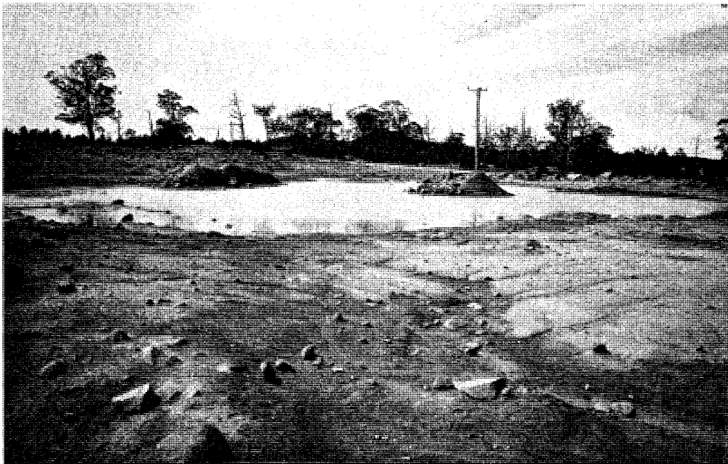
Extensive borrow pits alongside Arthurs Lakes Road; altitude 975 m; solifluction soil stripped for engineering purposes (1963-64) and not recolonised by vegetation due to lack of drainage and reclamation.
