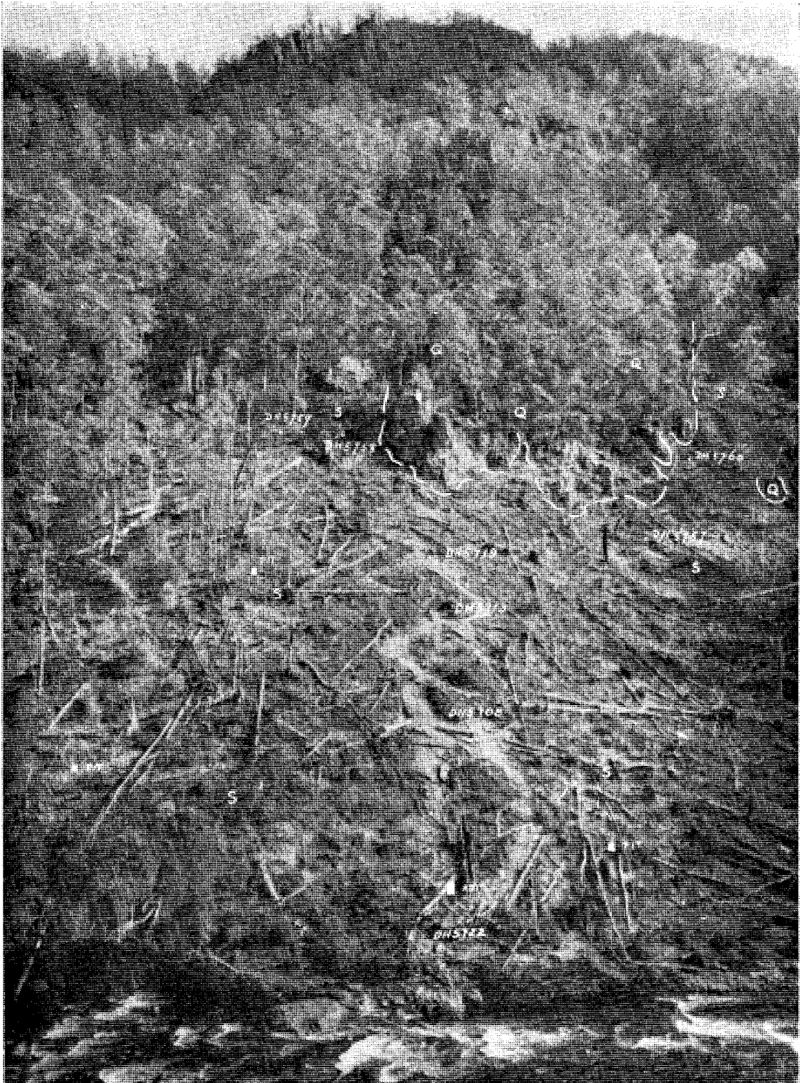
PLATE I.—The left abutment of Parangana Damsite showing cliffs of vertically foliated Precambrian Fisher Group quartzite (Q) and the talus slopes (S). The lower part of the talus covers glacial drift.
