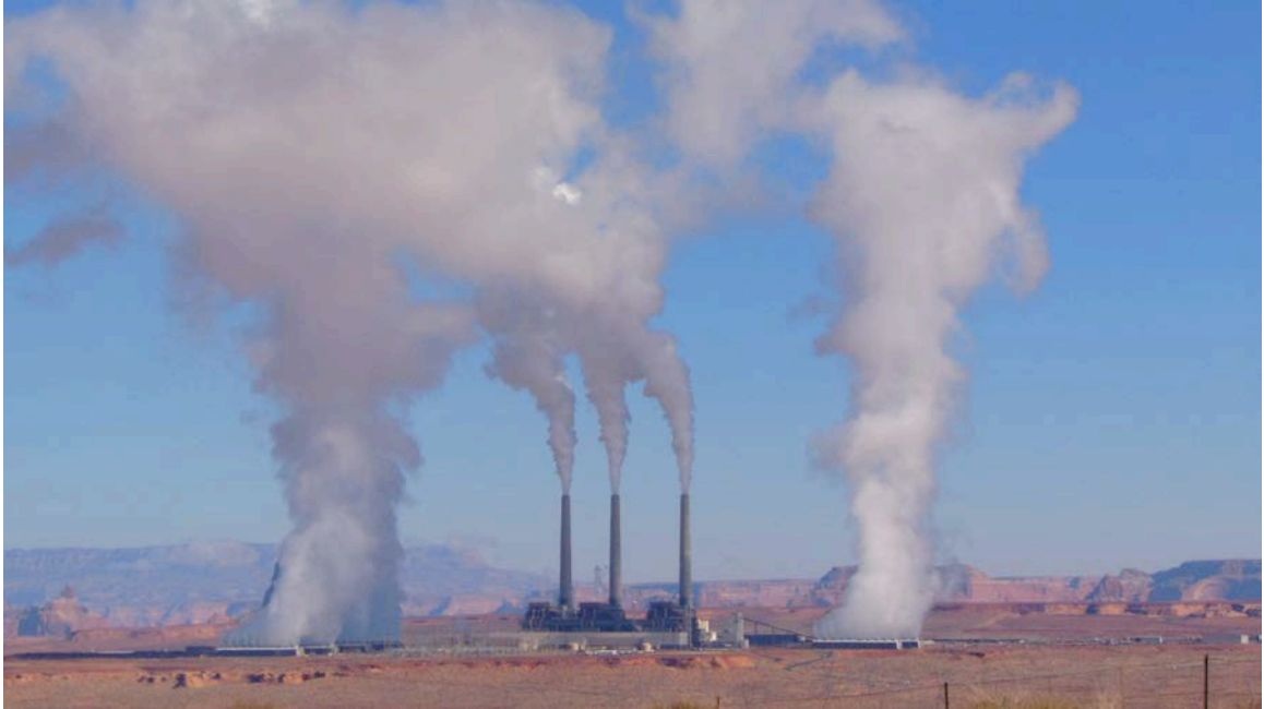
Figure 1: Navajo Generating Station, Page Arizona 2015. Photo taken by author.
