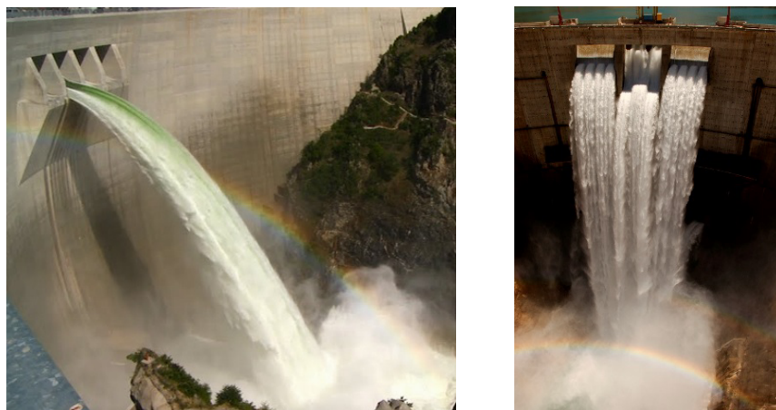
Fig. 1 Overfall spillways: Tsankov Kamak (BG) and Karun 5 (Iran)
