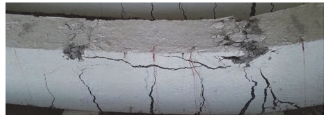
Figure 16. Crack pattern and failure mode of RC beam for copper slag 20% replacement and PP fibre 0,4%
