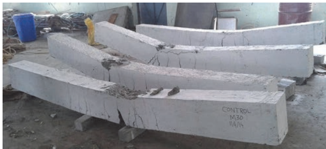
Figure 14. Reinforced concrete prototypes after testing
