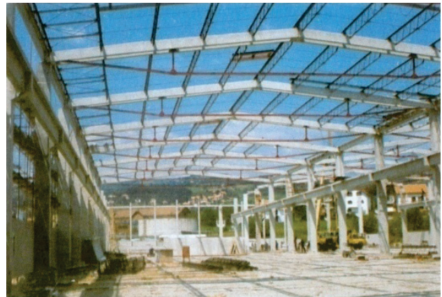
Figure 3 Industrial hall under construction
