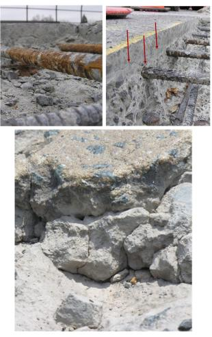
*Figure 1* Typical concrete bridge deck deterioration and damage: rebar corrosion (left), delamination (middle), and deck spalling (right).
