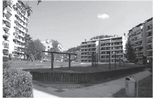
Figure 9 The Pilot Action Target Area Before Renovation
