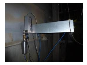
**Figure 2.** The analyser mounted on the wall of the boiler **Slika 2.** Analizator montiran na zid kotla
