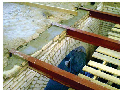
b) Reconstruction of brick barrel vaults above the basement
