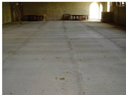
a) New full depth RC slab above the basement
