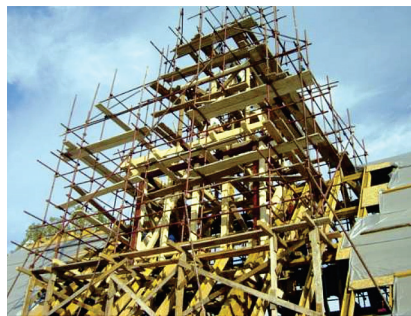
a) New timber structure of the tower
