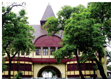
b) Northern facade with completed bays
