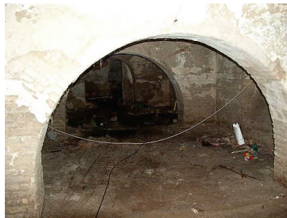
a) The basement prior to interventions
