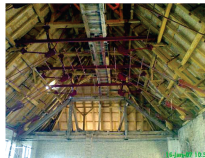
b) Reconstructed and repaired roof structure
