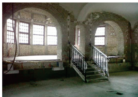
a) Internal appearance of the bays
