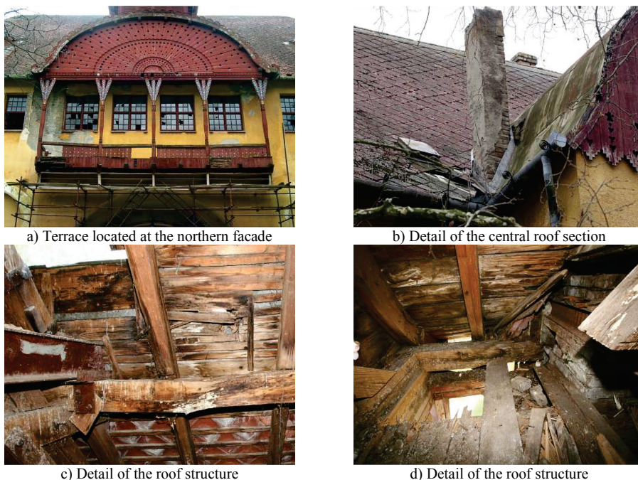
Figure 4 General condition of the roof
