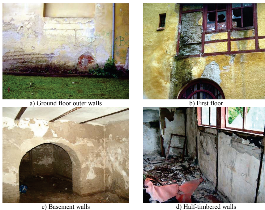
Figure 2 General condition of the walls
