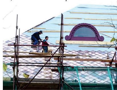
d) Copper plate roof finishing
