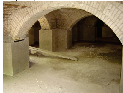
d) The basement after interventions
