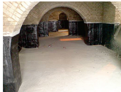
b) Waterproofing of the walls and floor of the basement
