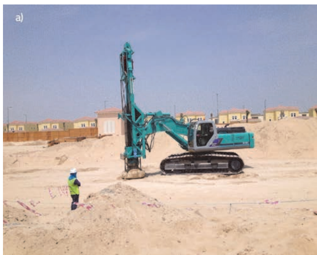
Figure 1. a) rapid impact compactor; b) impact foot with driving cap
