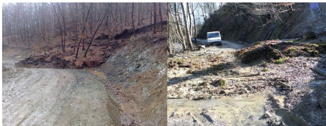
FIGURE 4. Left: Damages on forest road caused by landslide. Right: Damages on forest skid-trail
