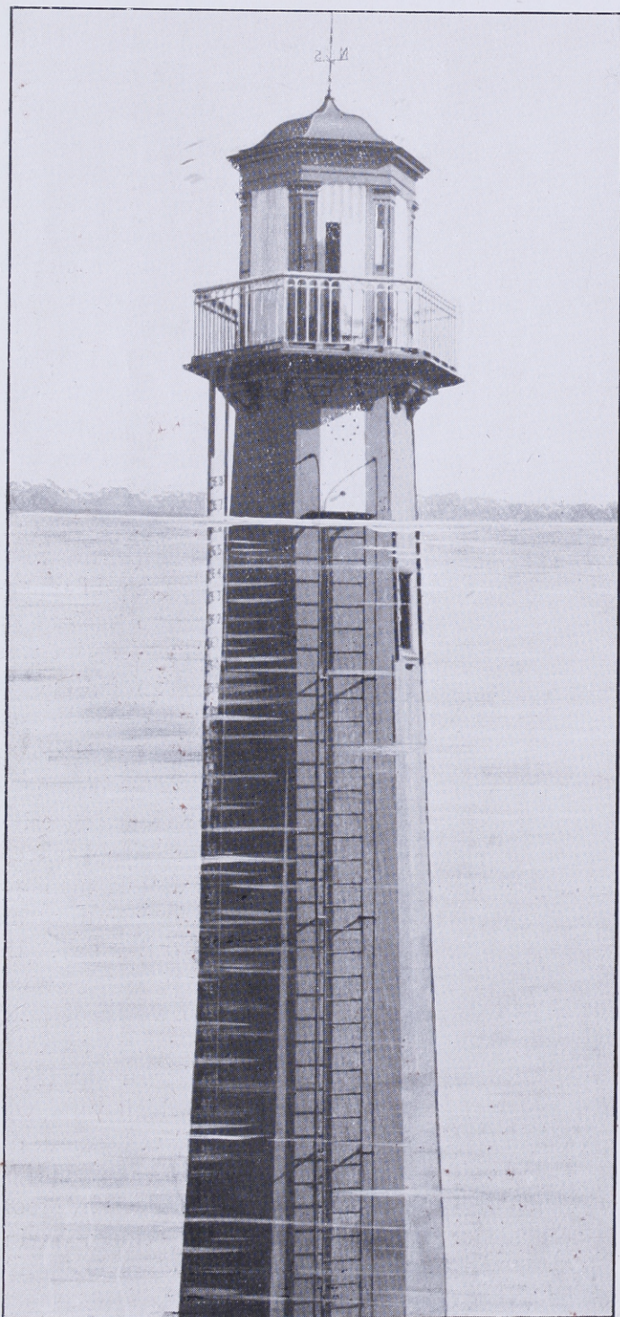
View of Valve Tower.
