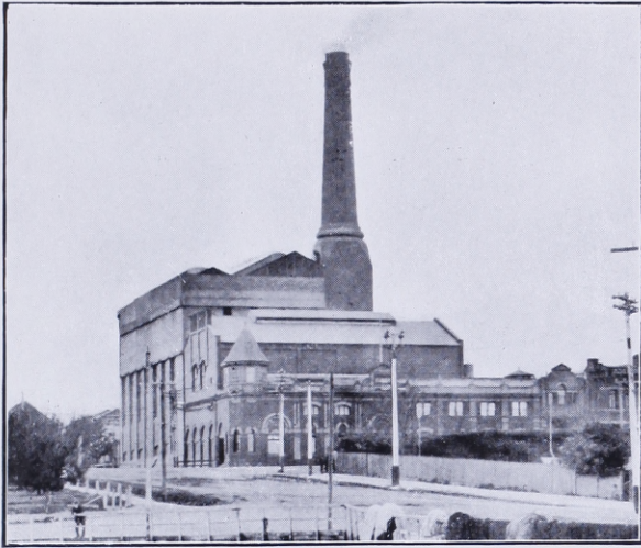
New Power Station.
