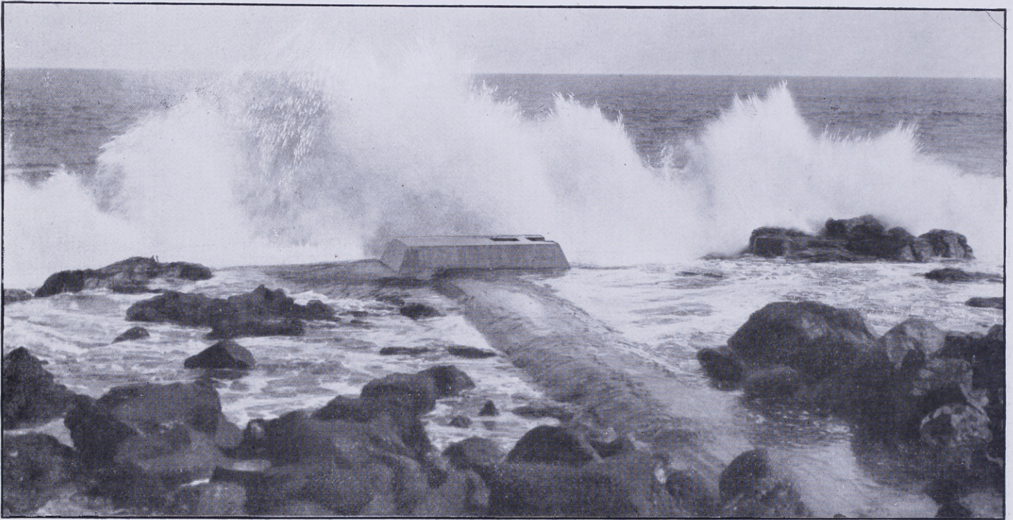
Outfall Sewer at Black Rock.
