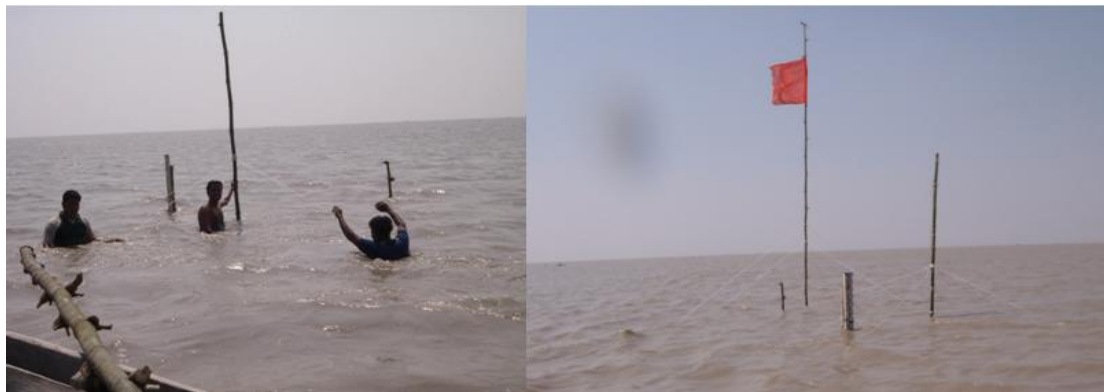
Figure 3. 3: Photo of installation of tide gauge in western offshore, 6 th March 2014
