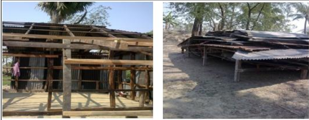
Figure 5. 12: Picture showing Re-built house (left) and Shifting house materials (right)
