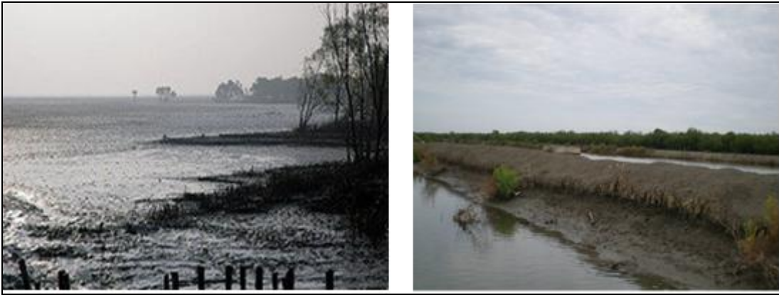
Figure 5. 11: Picture showing Bamboo revetment (left) and Heightening of dike (right)
