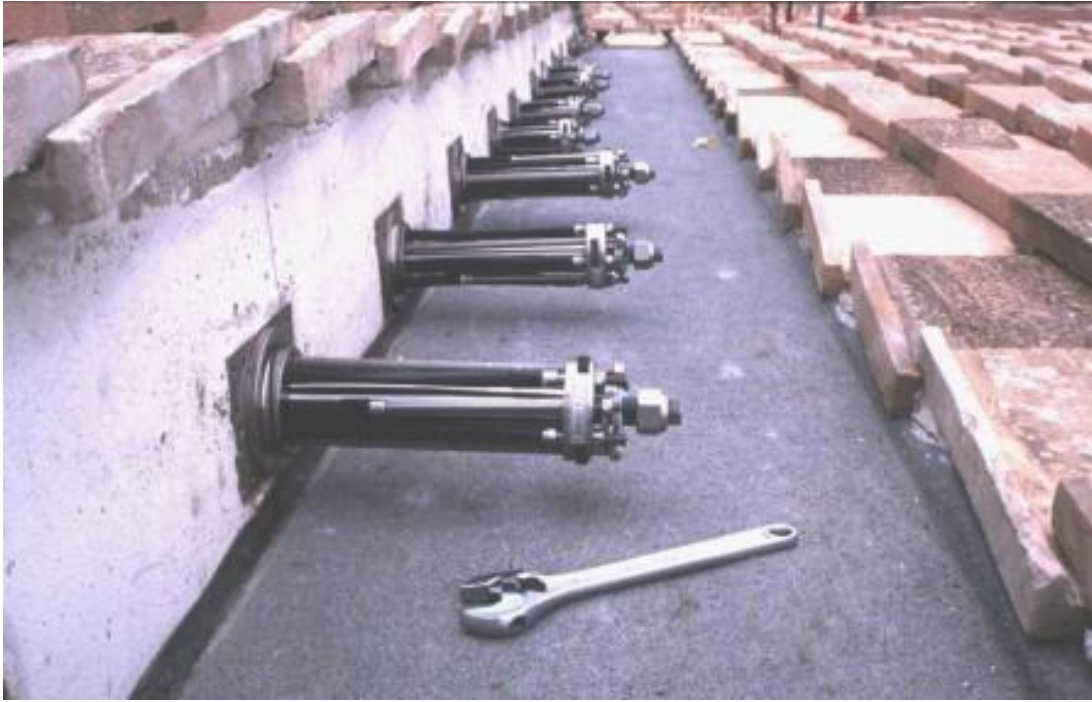
Figure 38 Picture of the entire SMA devices row at the end of the work.
