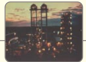
One of the largest refineries in Eastern Europe, the Gdansk Refinery has been a Honeywell customer for 20 years.
