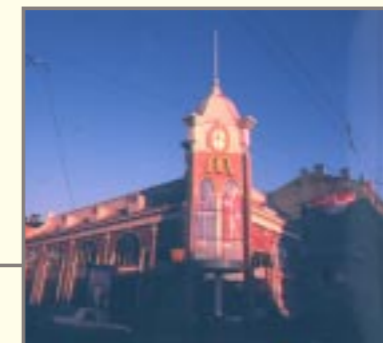
Honeywell fire and security and ventilation control systems are installed in most McDonald's restaurants in St. Petersburg and Moscow.
