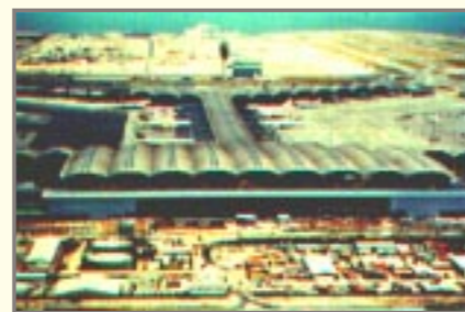
Honeywell Home and Building Control's mechanical building management system controls the fire alarm system, as well as security and access at the Hong Kong International Airport. (Photo courtesy of Hong Kong Airport Authority)
