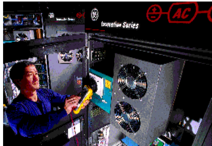
Ernest Linn of GE uses a multimeter to check the firing circuit on a new Innovation™ Series AC Drive, which provides customers with more power and reliability for their industrial processes.
