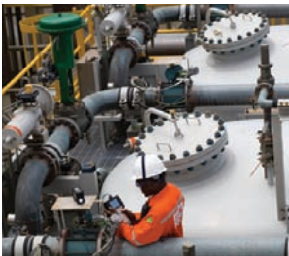
Onboard the Erha floating production, storage, and off-loading (FPSO) vessel, among the largest in the world, a technician conducts diagnostic checks.
