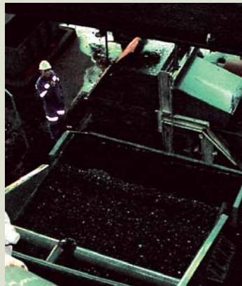
The coal discards washing plant at Anglo Coal South Africa's Goedehoop colliery has achieved an increase in coal recovery of 1.5%
