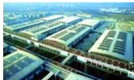
Shell Solar supplies additional power for the Munich Trade Fair Centre, Germany.
