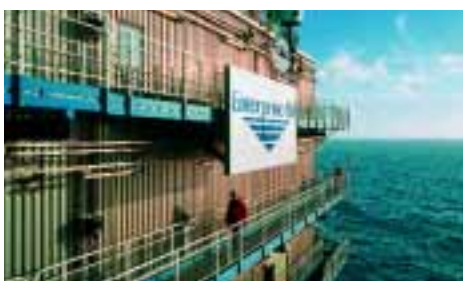
Enterprise Oil's Nelson platform in the North Sea.
