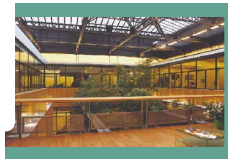
The Grenelle office building in Paris, a site based on HQE specifications.
