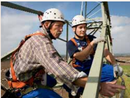
Some 7,000 employees take care of RWE Energy’s line maintenance
