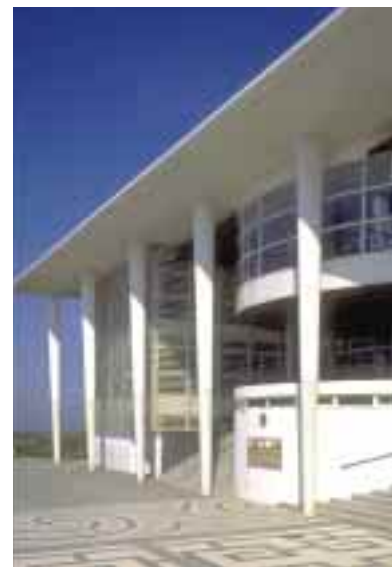
FRANCE LAFARGE CIMENTS At Sausset-Les-Pins high school (Bouches du Rhône), super-white cement was used in the concrete for the architectural pre-cast units elements such as the columns and facade.
