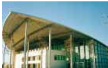
SPAIN LAFARGE ASLAND High-strength cement was used in the construction of the Valence Conference Center, and rapid-setting cement used for the pre-cast roof elements. The building was designed by British architect Norman Foster.
