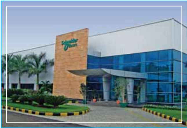
Accessing and monitoring energy data digitally has enhanced efficiency improvements at the Schneider Electric Hyderabad plant in India.
