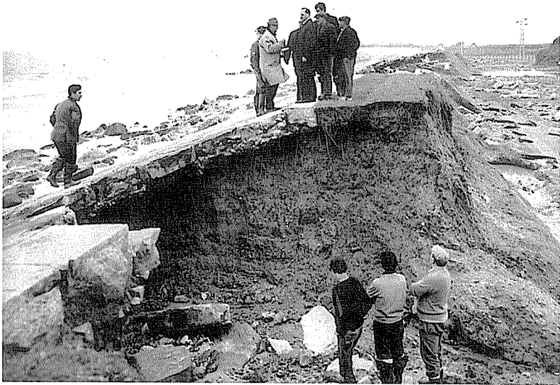
Fig. 4 Destruction of the "murazzi" at Pellestrina, after the very violent storm of 4 November 1966 (Courtesy of Cameraphoto, Venezia).
