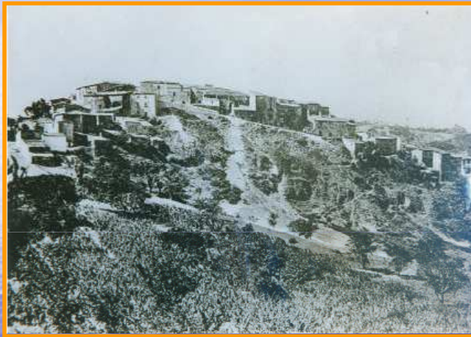
Old Aquilonia, Landslide
