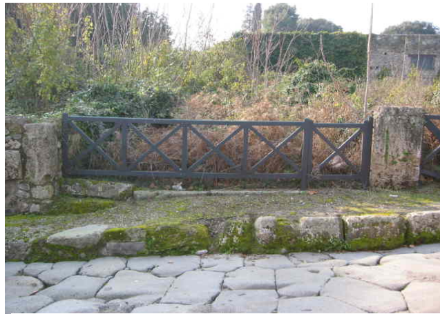
Fig. 4. The shop at VIII.7.9-10, prior to investigations
