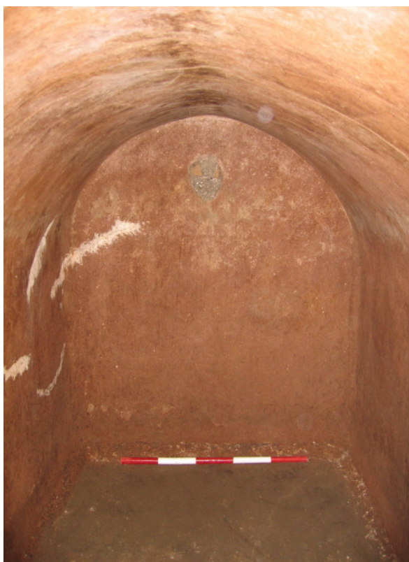
Fig. 15. Southern end of the cistern. Note the patching on the wall at left
