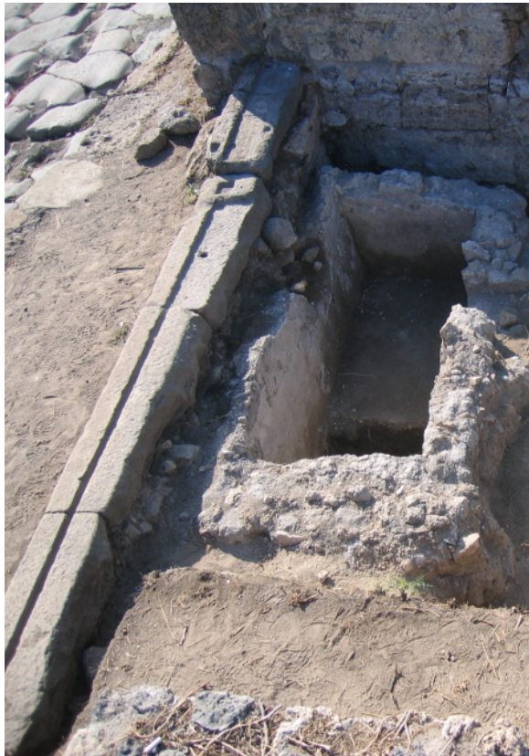
Fig. 6 Large rectangular tank inside the threshold. Note the two separate entrances to the property: a wide retail opening together with a narrower entrance (at top of photo) to a possible flight of stairs
