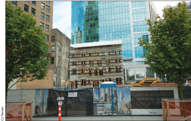
Figure 2. As aging urban infrastructure degrades, many ecological, social, and economic problems, as well as opportunities, may arise. Urban ecologists will be called on to help develop science and policy to maximize the opportunities for urban inhabitants equitably and in sustainable ways.
