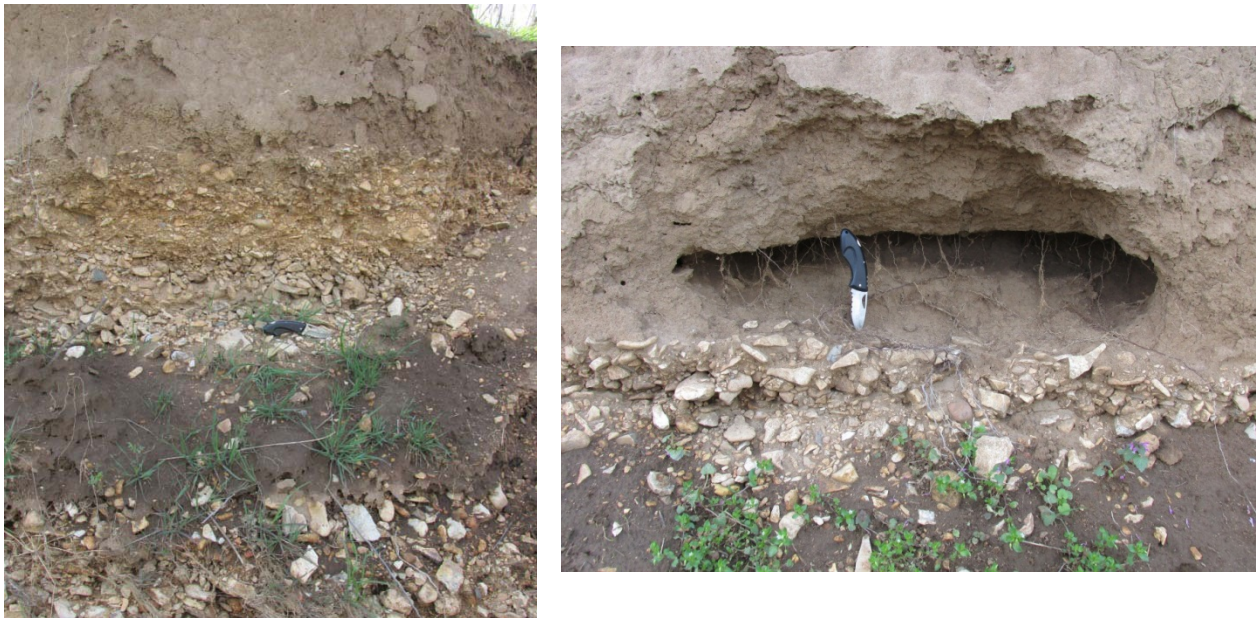
Figure 2. Streambank at the Barren Fork Creek field site including the bank profile (left) and a seepage undercut (right). Note the sloughed material in the bottom of each picture from recent bank failures. These complex alluvial deposits include both clean gravel lenses associated with rapid flow and transport (left) as well as fine gravel lenses that can cause lateral flow and seepage erosion.
