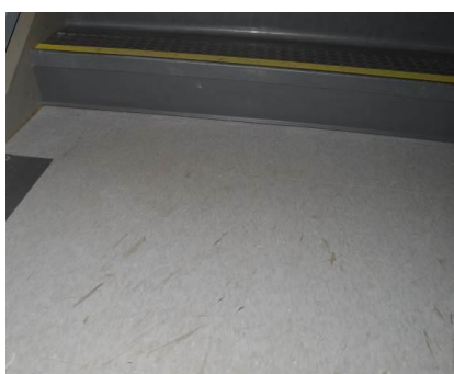
Figure 5.1.1 D: Site D – View of VCT Floors in Stairwell
