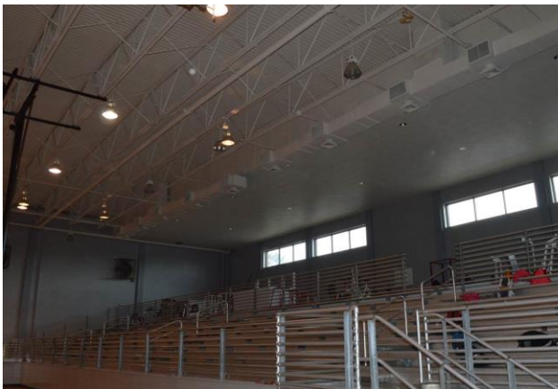
Figure 5.2.1F: Site B – View Gymnasium From Entrance
