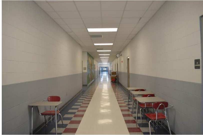
Figure 5.2.1I: Site B – View from English Wing Hallway into Main Building Hallway
