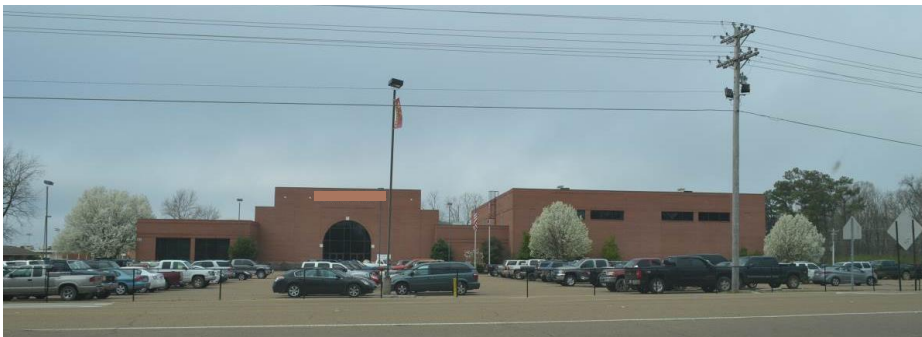
Figure 5.2.1A: Site B – Front Exterior Façade
