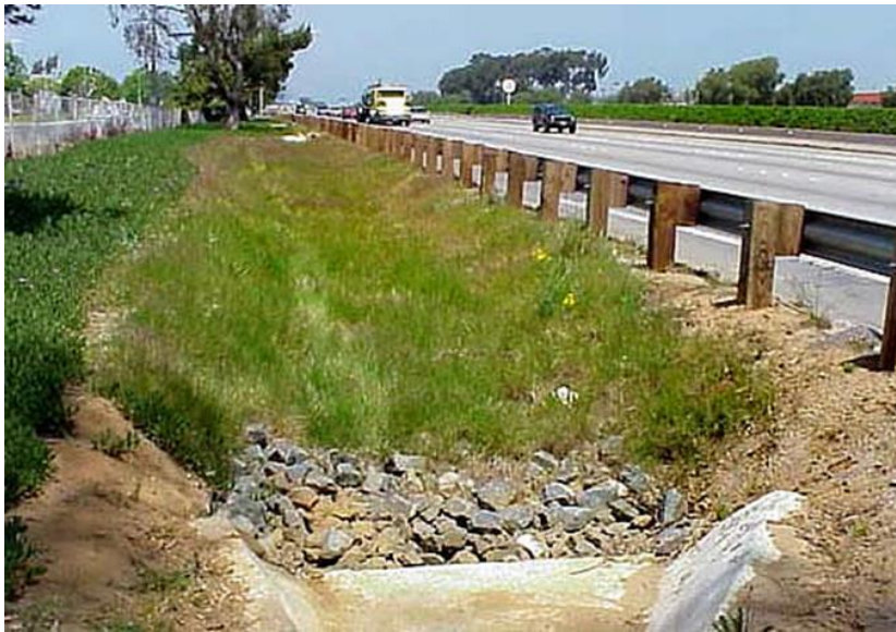
Figure 3. 14 Grass lined swale (Bioinfiltration Swales)
