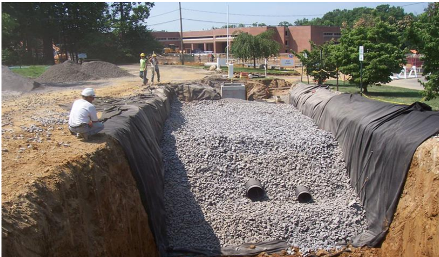
Figure 3. 13 Infiltration Trench (DCCC 2009)
