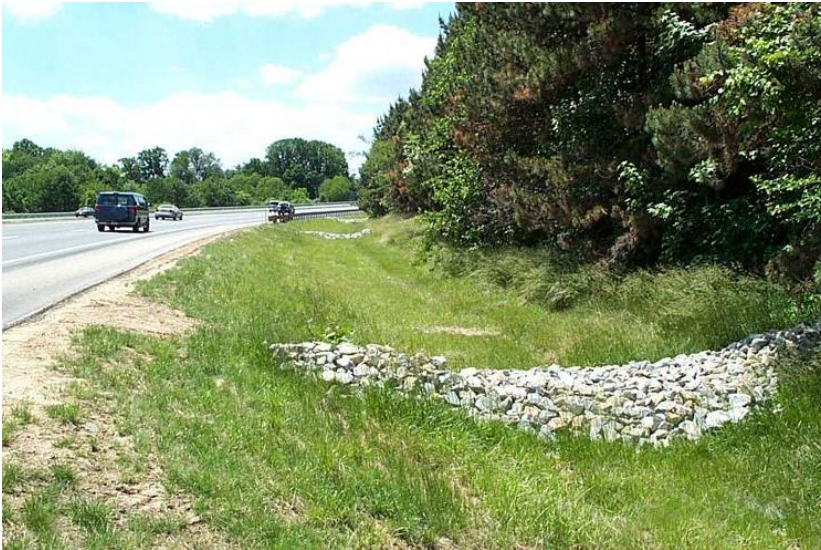
Figure 3. 15 Grass lined swale with rock check dam (DDOT 2014)
