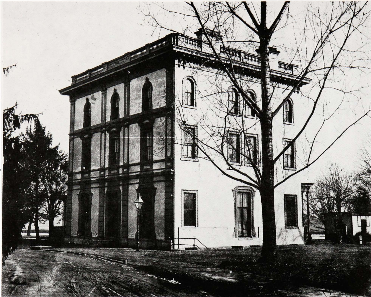
Academic Building, Washington Barracks (now Ft. McNair) in 1902, first home of the Board of Engineers for Rivers and Harbors.
