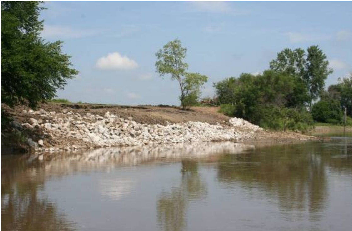
Figure II.3.7. Photograph from July, 2008 of sloughed bank looking upstream.
