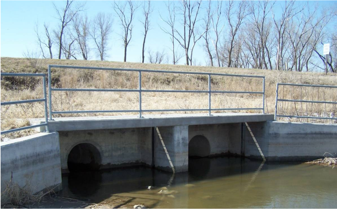
Figure III.1.42. Photo of the Tieville Bend outlet structure during pump operation to facilitate fish movement.
