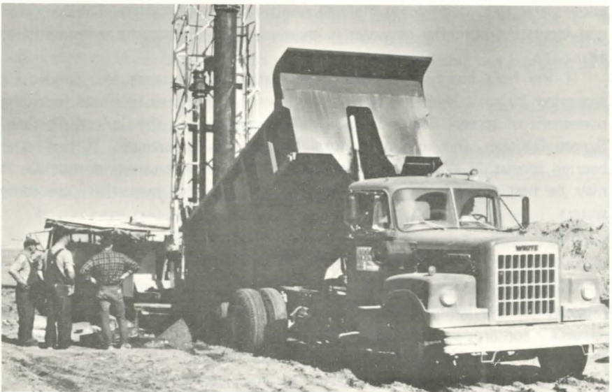
Figure 3. Well screens must be matched to the gravel pack material. In general, most slots are too wide.
