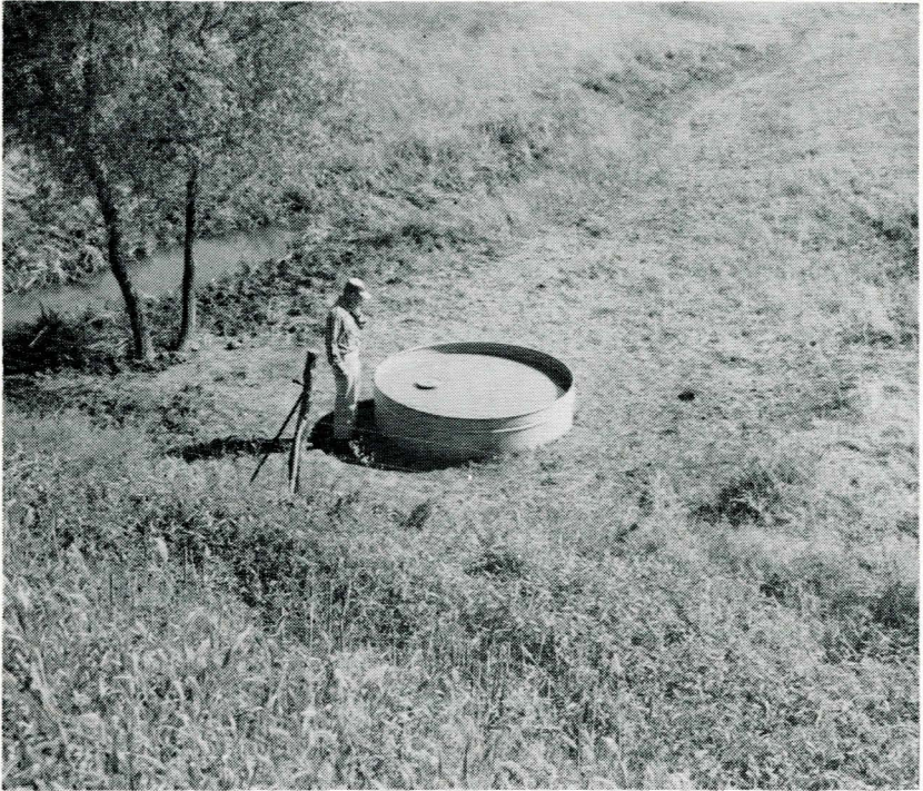
Stock tank with float and valve below fenced reservoir.
