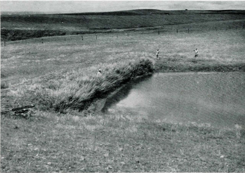
Stockwater reservoir showing willow rip-rap on face of dam to protect against wave action.
