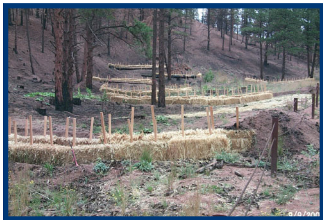
Figure 10.3 —Straw bale check dams placed in channel by the Denver Water Board after the Hayman Fire, 2002, near Deckers, CO. (Photo by Peter Robichaud).
