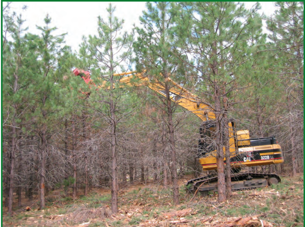
Figure 8.11. Rotary head masticator (boom-mounted) effectively shredding single trees.
