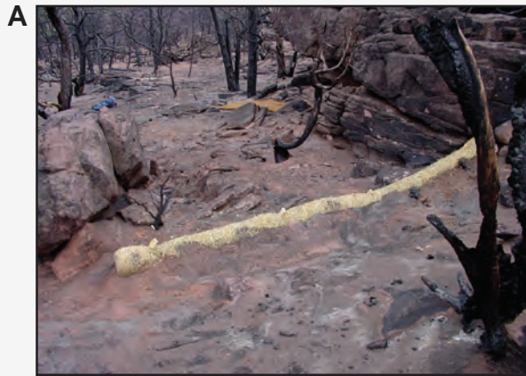
Figure 9-S4.a —Burned Area Emergency Rehabilitation work to protect a rock shelter following the 2002 Mustang Fire, Ashley National Forest, Utah. Straw wattle (foreground) was used as a runoff barrier to protect the rock shelter from water coming in from the side, which could result in erosion damage. An erosion blanket (brown patch in mid-ground) was used to protect the floor of the rock shelter from water flowing off of the overhanging ledge (Johnson 2004a,b) (photo August 2002, by Clayton Johnson, USFS Ashley National Forest).
