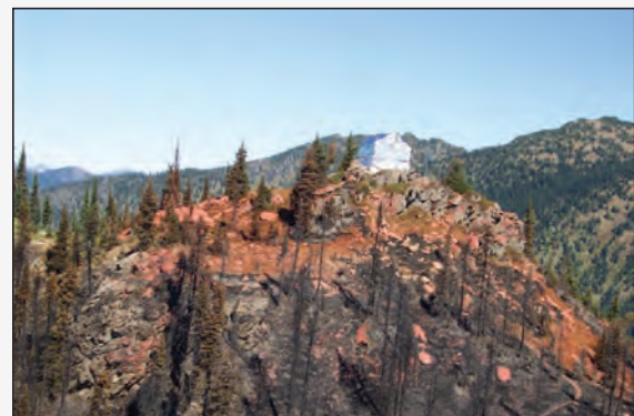
Figure 9S-5g —Little Snowy Lookout following foil-wrapping and pretreatment with aerial retardants.
