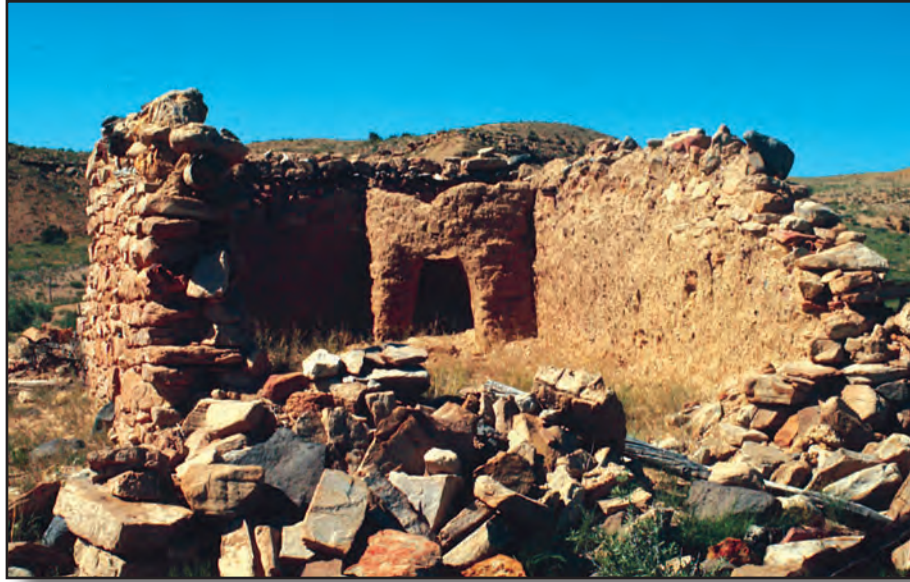
Figure 6-1 —19 th century Hispanic structure, New Mexico; constructed of sandstone, adobe plaster, and log roof beams.
