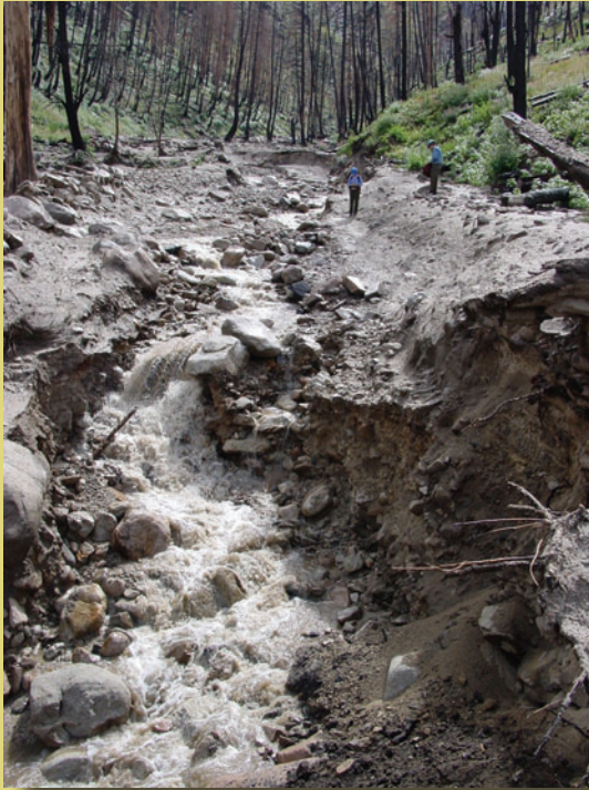
Figure T3-3: Steel Creek debris flood following the Hot Creek Fire.
