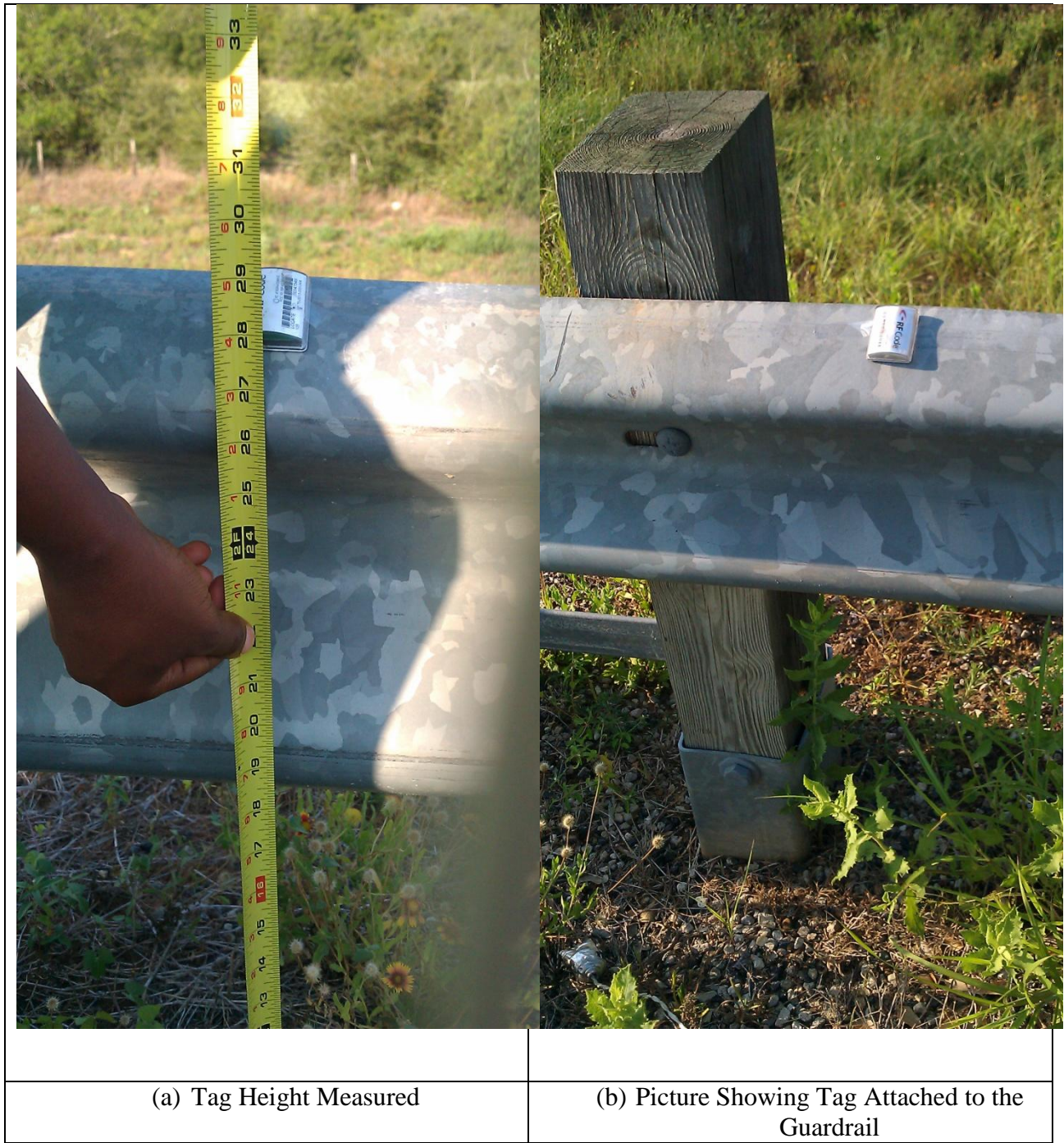
Figure 4.9 Tag Attached to a Guardrail for Dynamic Testing
