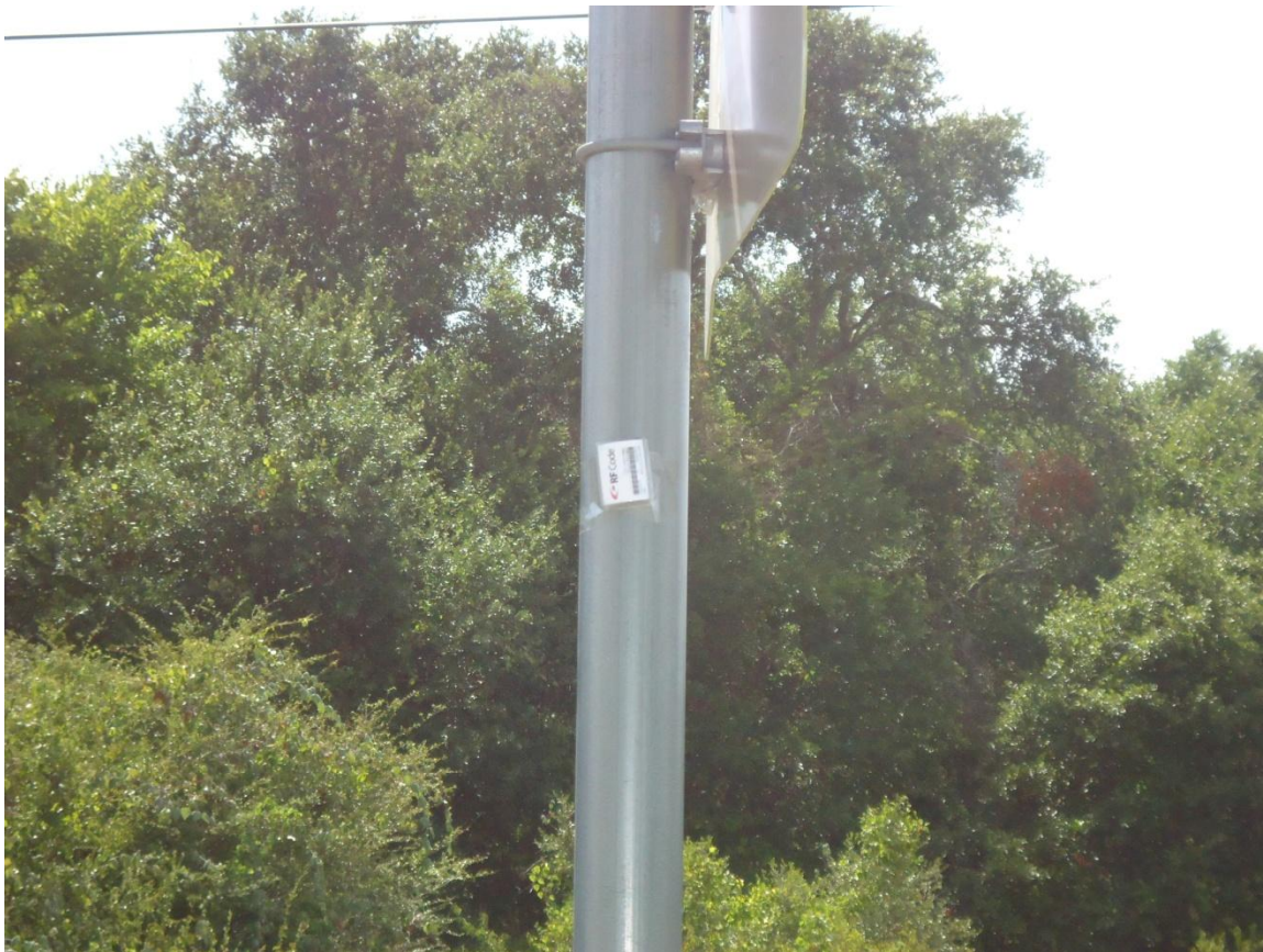
Figure 4.7 Tag Attached to a Signpost at 7 ft
