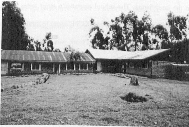
Figure 6.5: Eskuru Secondary School
