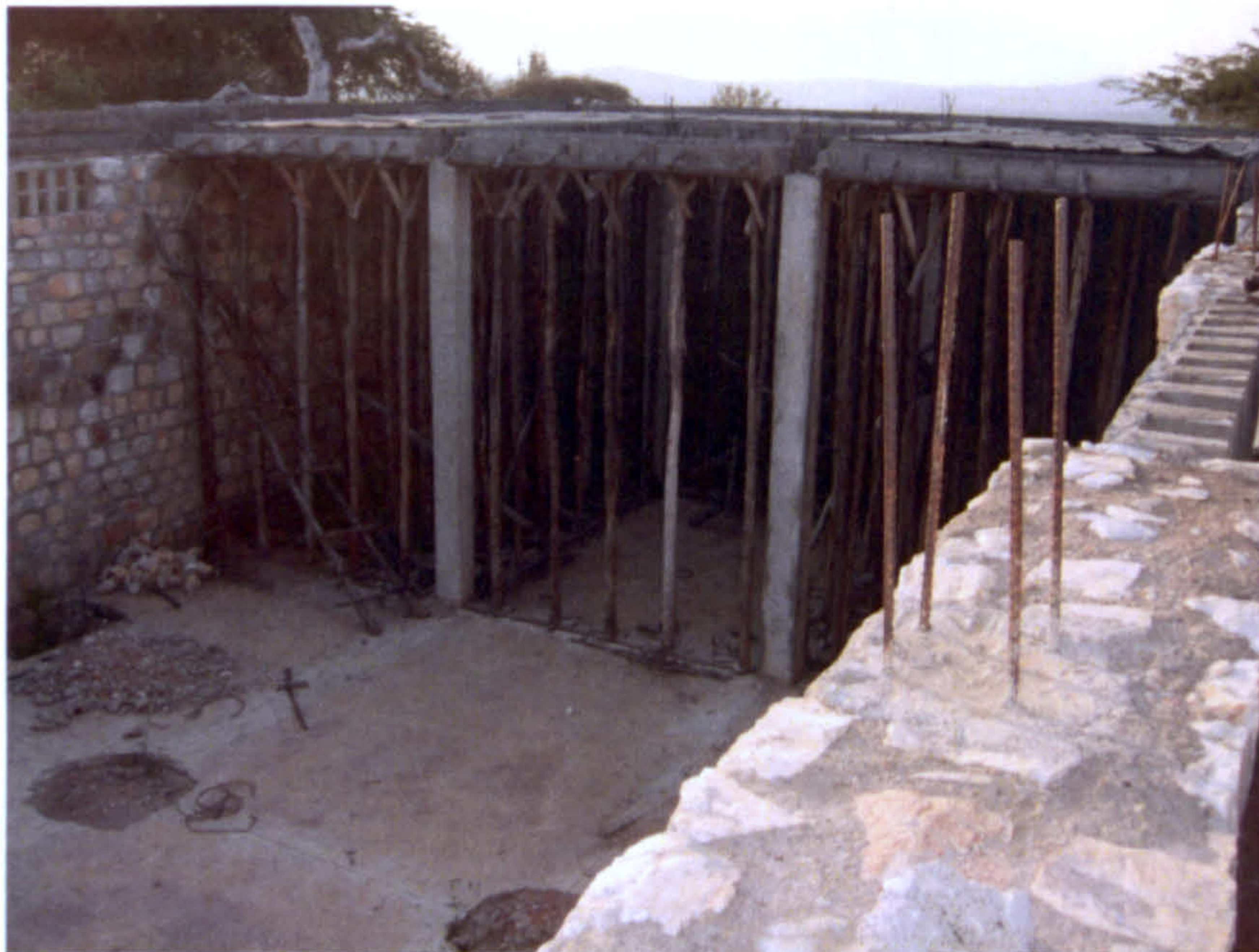
Mugina: new genocide memorial site under construction, August 2006
