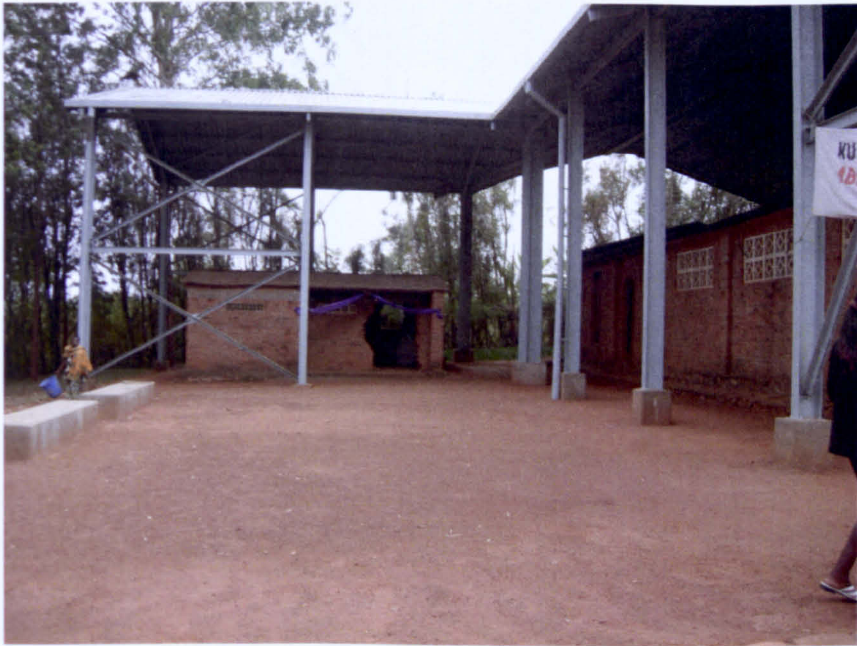
Ntarama genocide memorial: new roof, August 2006
