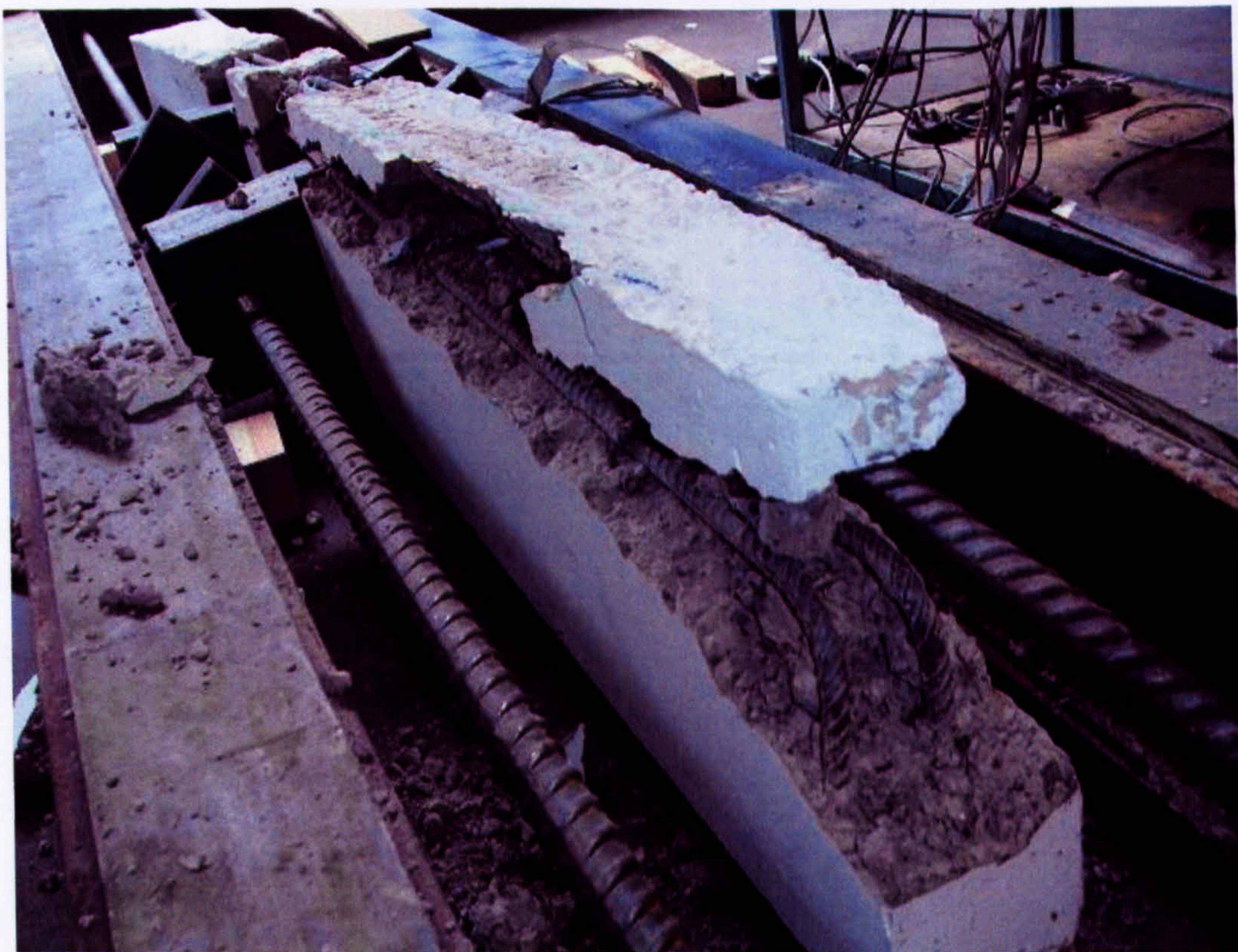
(b) B2 (fracture of end concrete block)
