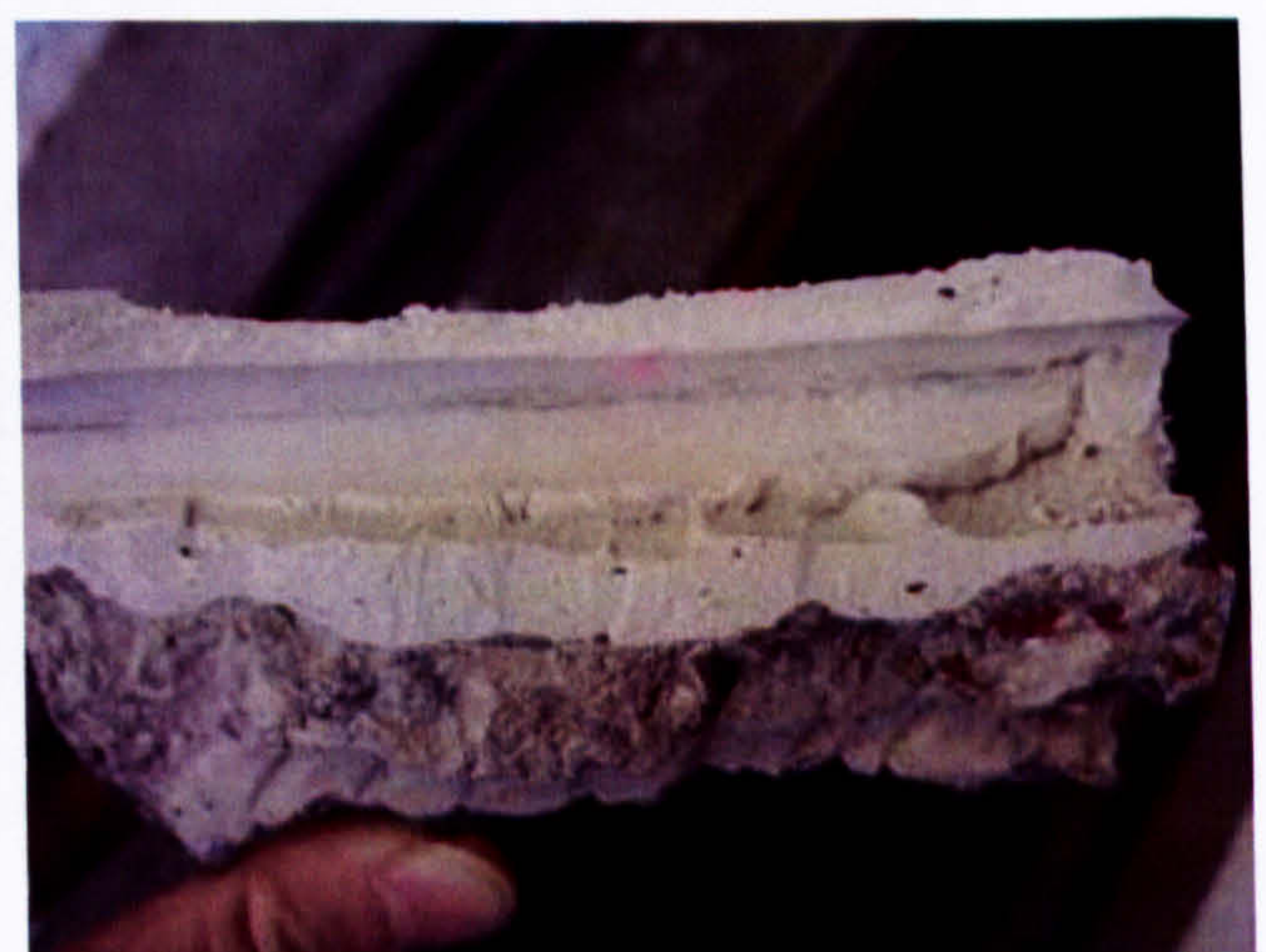
(b) Block of concrete after fracture
