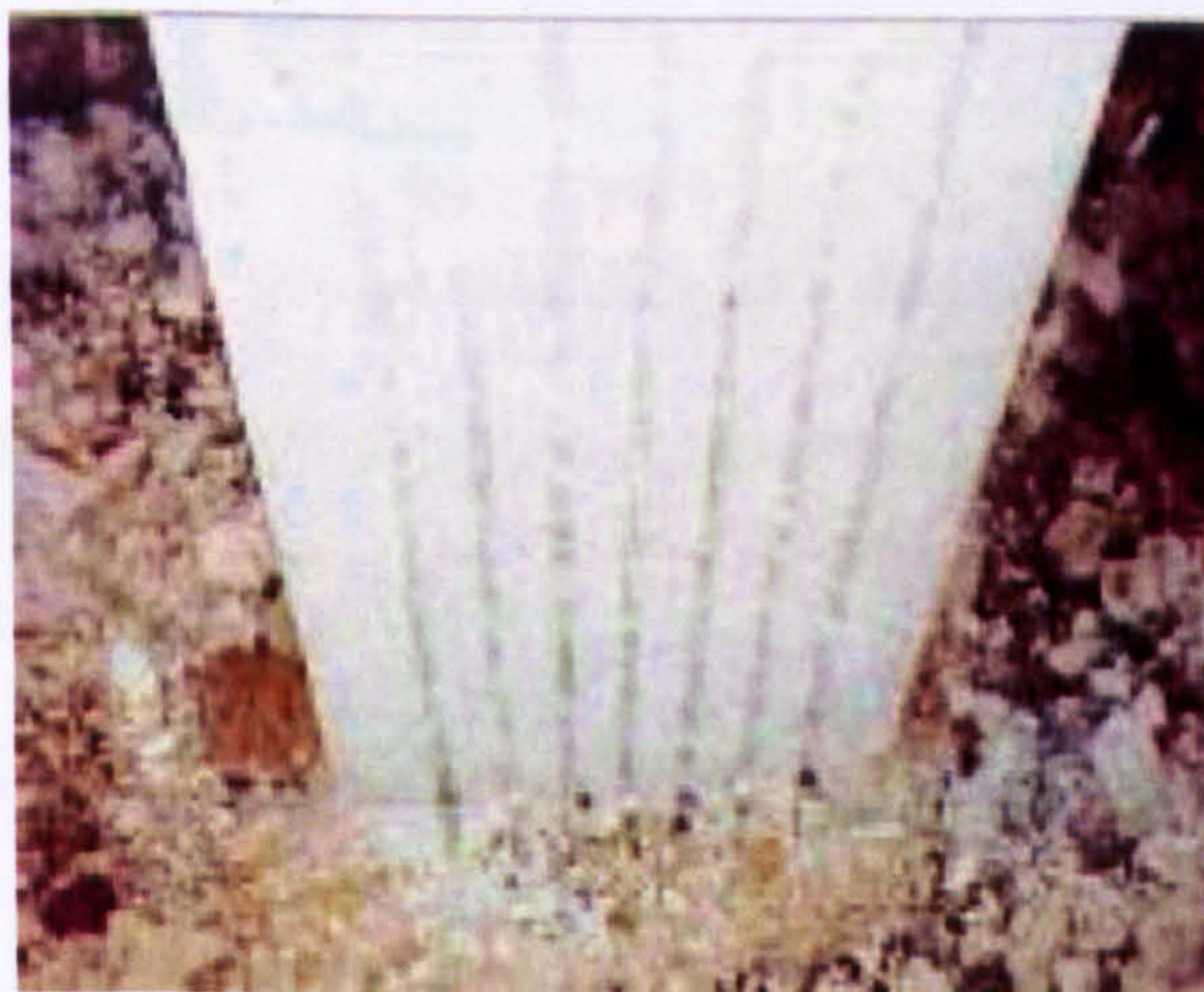
(c) Strengthened Bridge in service (Alkhrdaji et al. (1999))
