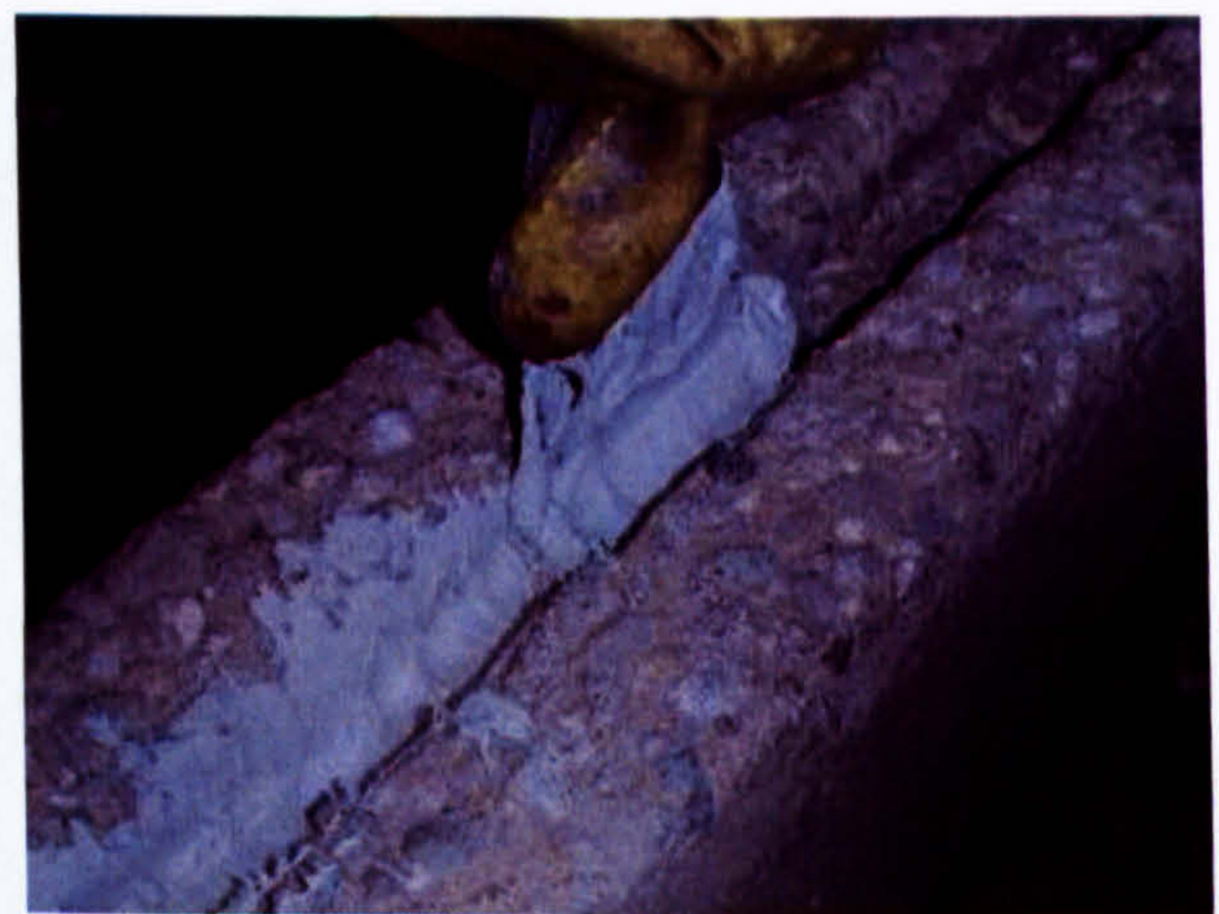
(b) Half fill the groove with epoxy
